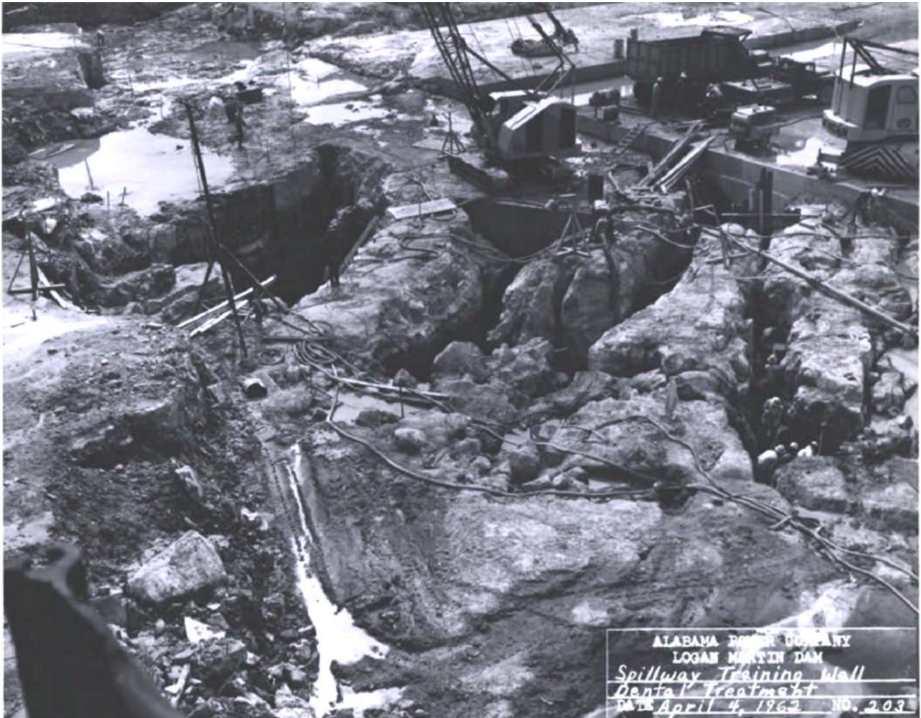
Figure 3. Well Developed Solution Features Revealed During Construction
