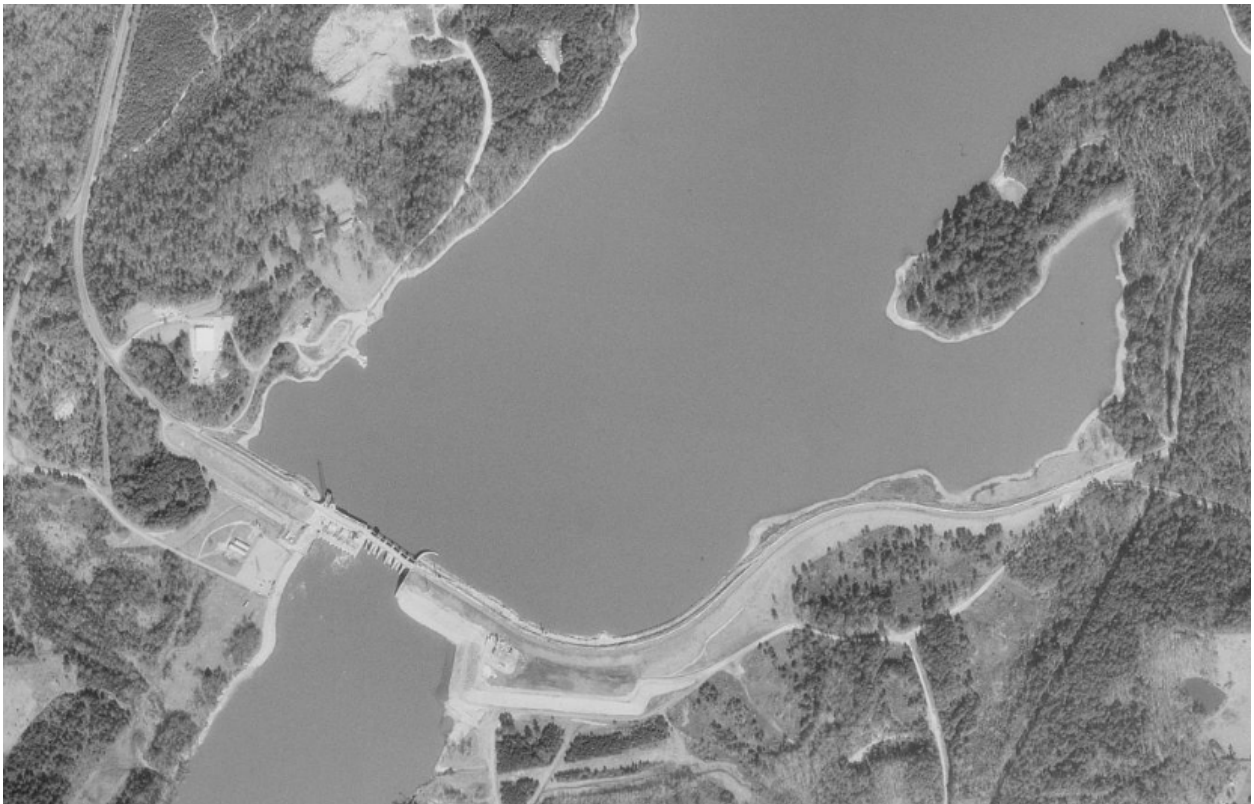
Figure 2. Aerial View of Logan Martin Dam
